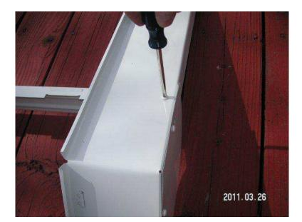
Use bolts and nuts to attach ends of bottom panels to underside of header.
