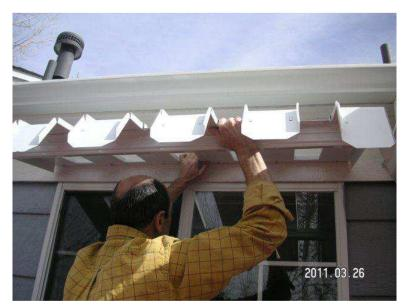
Drill a hole (11/64" bit) in the underside of runner for each of the left and right end rods and attach each end rod to underside of runner with a bolt and nut.
