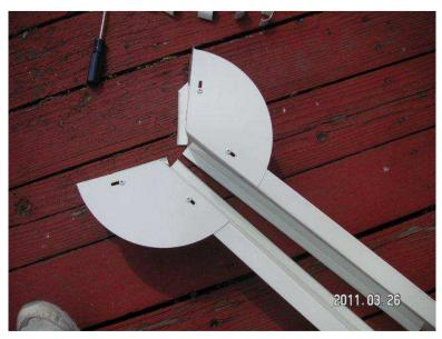
Attach left end panel to end of header with bolt and nut.
