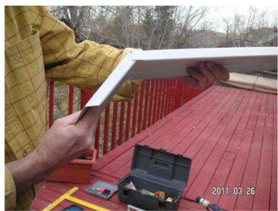
Slide top panels on top of gaps between bottom panels.
