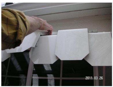
Lock valance parts of top panels using slots in bottom panels.
