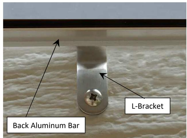
17. Install an L-Bracket under the center of each Back Aluminum Bar for an additional support.
