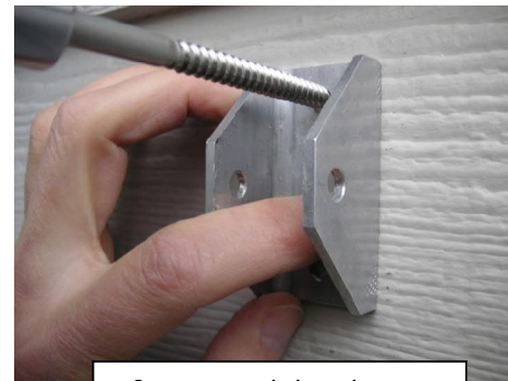
Secure each bracket to wall with two fasteners
