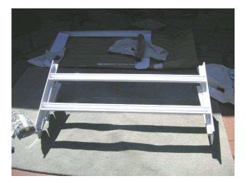
Attach left and right end pans to the flashing through holes provided in pans and flashing using the  $\#8-32 \times 1/2$ " bolts and #8 nuts.
