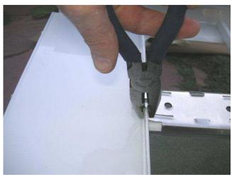
Bend down the valance parts of top covers, snap the covers over the clips and slide them back toward the flashing. (Top pans may be installed after the awning is hung.)
