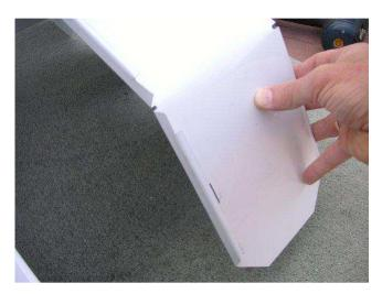
Position the apron bar behind the bottom pans and secure it temporarily with pieces of cardboard or paper to hold it in place.
