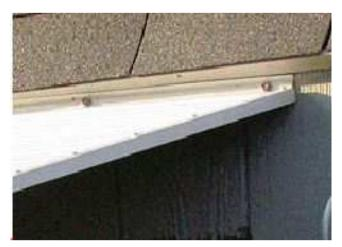
Attach the front of support arm with a self-tapping screw through the pre-drilled hole to the underside of side rail on each side.
