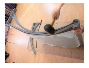
7. Install one of the brackets. Use a rubber mallet if necessary.
