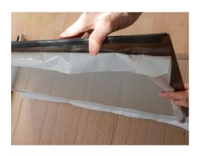
3. Install a rubber seal on the long side of the PC sheet. It is easier to install when the PC sheet is positioned vertically.
