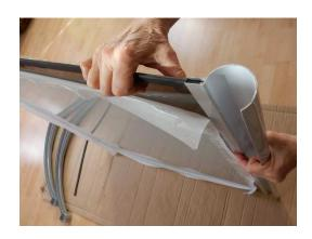
6. Stand the PC sheet on the short side and install a short rubber seal.
