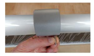
Secure the additional section's front gutter in the connecting bracket by drilling a pilot hole through the bracket and the front gutter and driving a small screw into the front gutter as shown.
