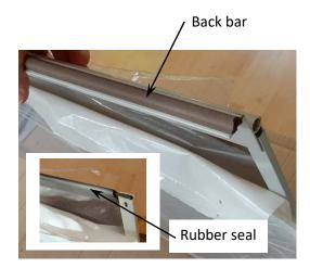
8. Install a rubber seal on the back edge of the PC sheet, then install the back aluminum bar. The flat side of the back bar should be on the side of the non-transparent protective film. It will face up when the awning is installed.
