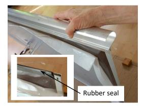
Install a rubber seal on the front edge of the PC sheet, then install the front gutter. The open side of the gutter should be on the side of the non-transparent protective film.
