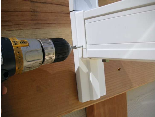
28. Secure the middle and bottom T-bracket covers with self-tapping screws.
