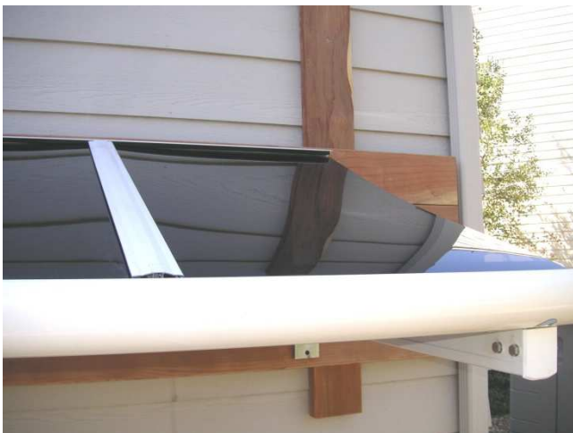
18. Insert the right side polycarbonate sheet.
