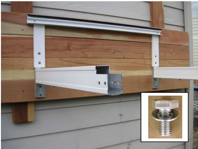
6. Attach projection beams to the T-brackets using 4 bolts with washers for each beam.
