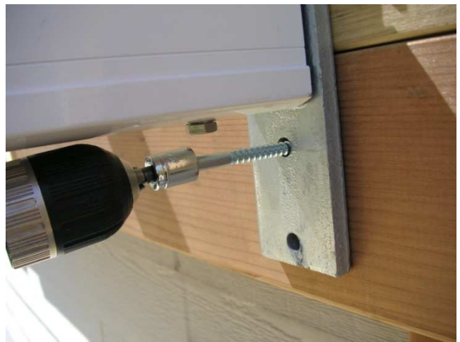
25. Drill pilot holes and secure the T-brackets through remaining holes in each T-bracket using appropriate fasteners.
