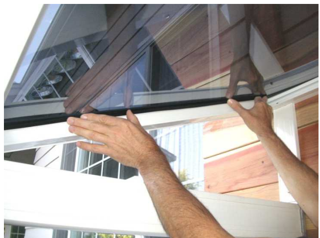
21. Insert rubber strips along the sides and back of each polycarbonate sheet. Each rubber strip section does not have to be in one piece.
