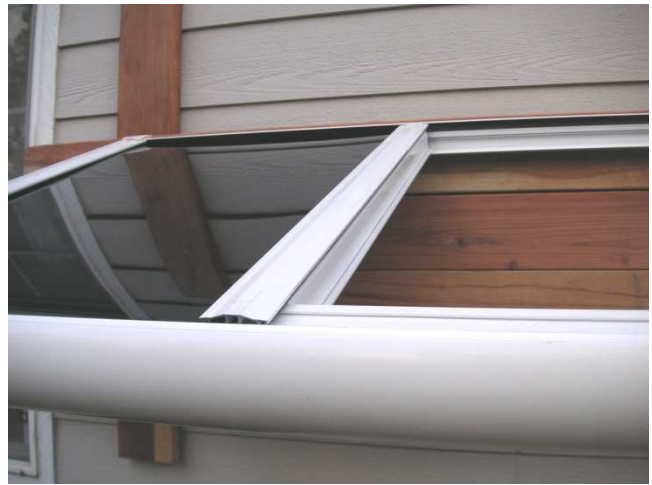
17. Install the middle rafter. If your awning has more than one middle rafters, install remaining middle sheets and middle rafters.
