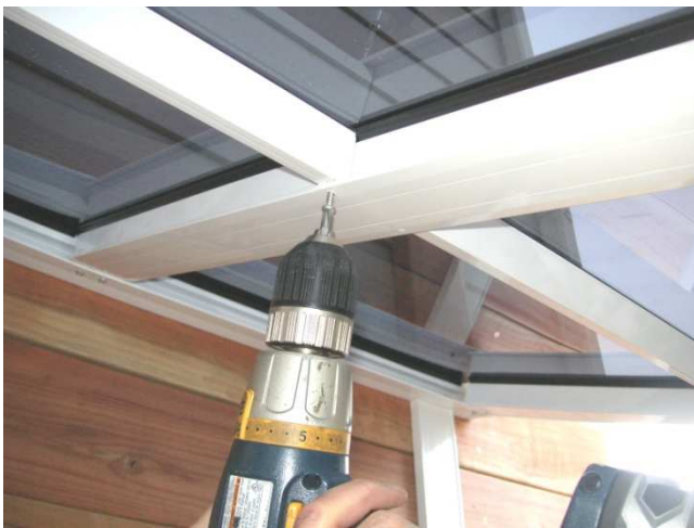
24. Secure polycarbonate sheet middle supports with self-tapping screws.
