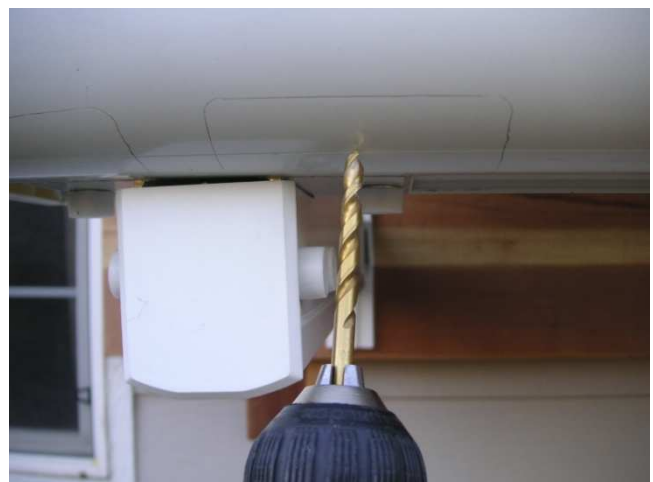
31. Drill several small water drainage holes in the center of the marked area or, if the downspout is not used, drill holes in the desired water drainage location.
