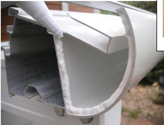
12. Apply caulk along the inside edge of the gutter on the left side.
