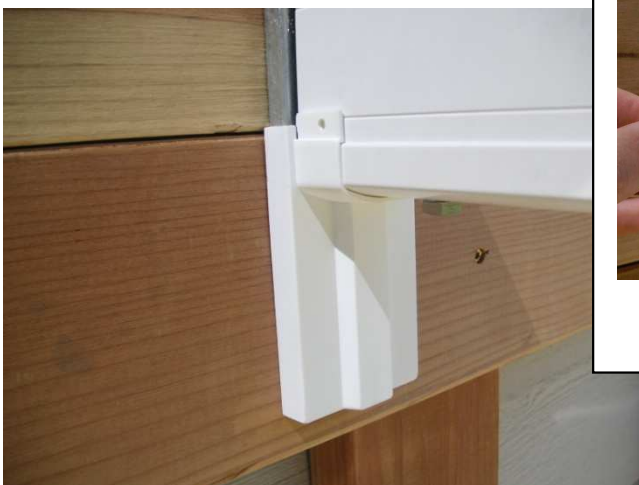
26. Install the bottom T-bracket covers.
