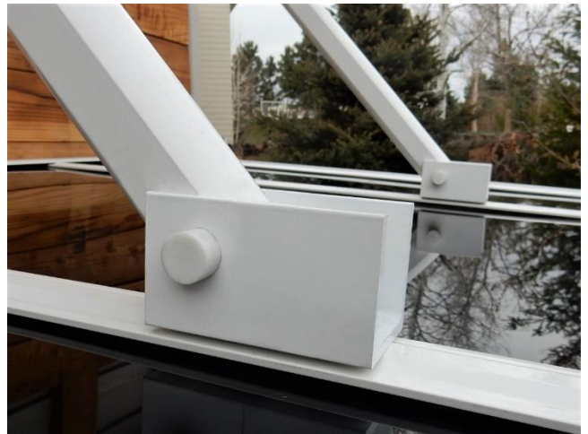
21. Tighten all nuts and install bolt and nut caps.
