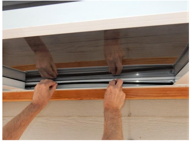
19. Insert rubber strips along the sides and back of each PC sheet. Each rubber strip does not have to be in one piece.
