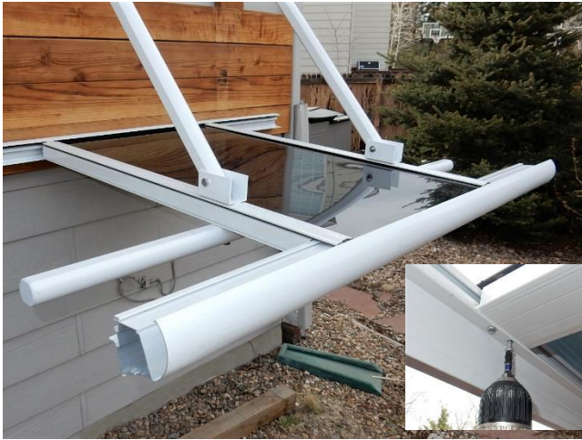
12. Attach the gutter to the middle rafters using self-tapping screws.
