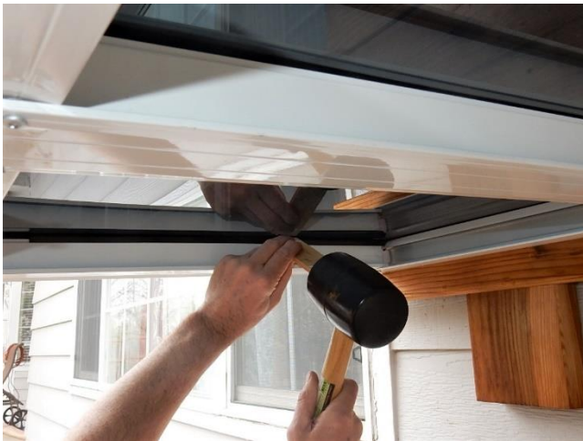
20. Drive the rubber strips in with a mallet and a piece of soft material, such as wood.
