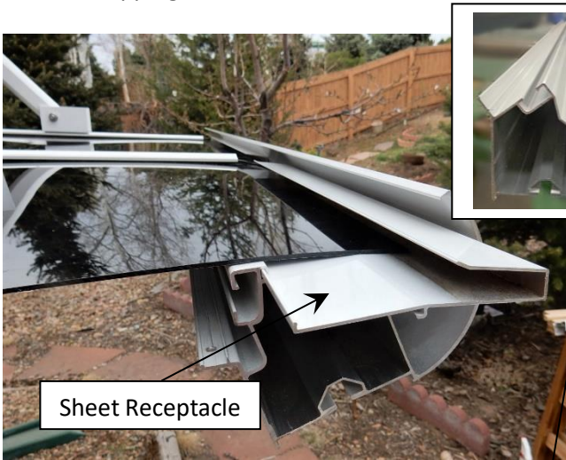
14. Insert the sheet receptacles, one for each PC sheet. (Skip this step if your gutter has a built-in sheet receptacle similar to the one shown here.)
