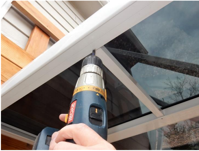
18. Install PC sheet middle supports and secure with self-tapping screws.
