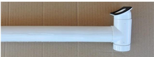
22. To use the optional downspout, assemble the water receptacle with the horizontal drain pipe using caulk to seal pipe connection.
