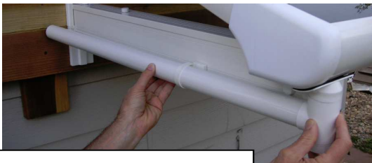
Alternative drain pipe locations
