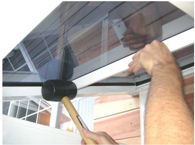
23. Install polycarbonate sheet middle supports and adjust their positions using a mallet.
