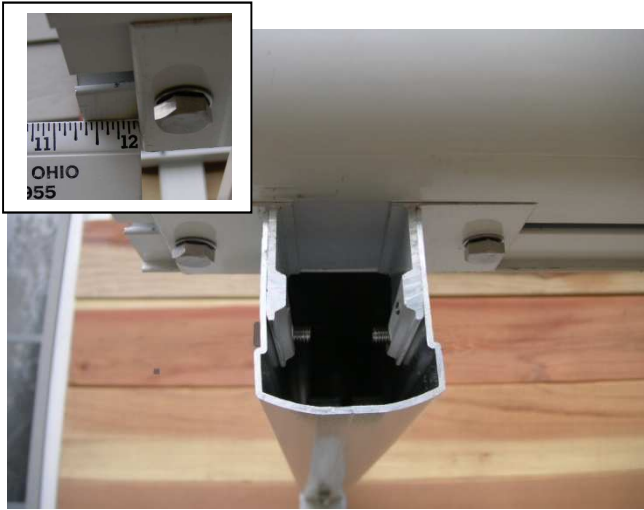
10. Attach the gutter to the supports using 2 bolts with washers for each support. The supports should be positioned at least 5/8" in from the ends of the gutter.
