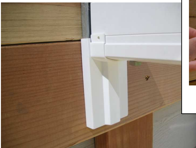
26. Install the bottom T-bracket covers.
