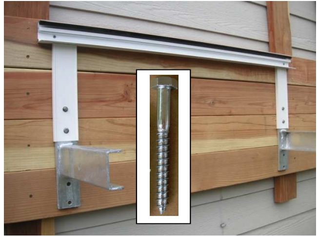
5. Use appropriate heavy duty fasteners to attach the T-brackets and their top covers.
