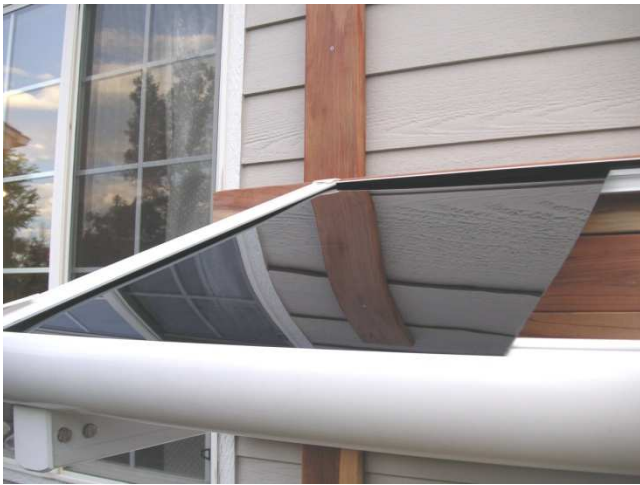
16. Insert the left side polycarbonate sheet.
