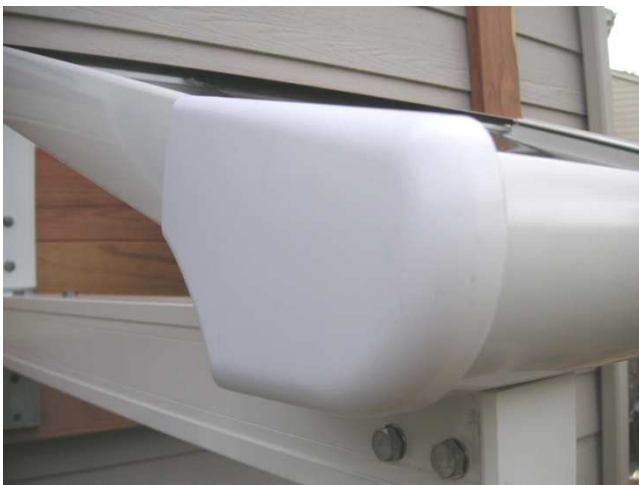
14. Install the left edge rafter with caps.
