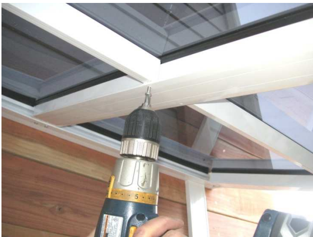
24. Secure polycarbonate sheet middle supports with self-tapping screws.
