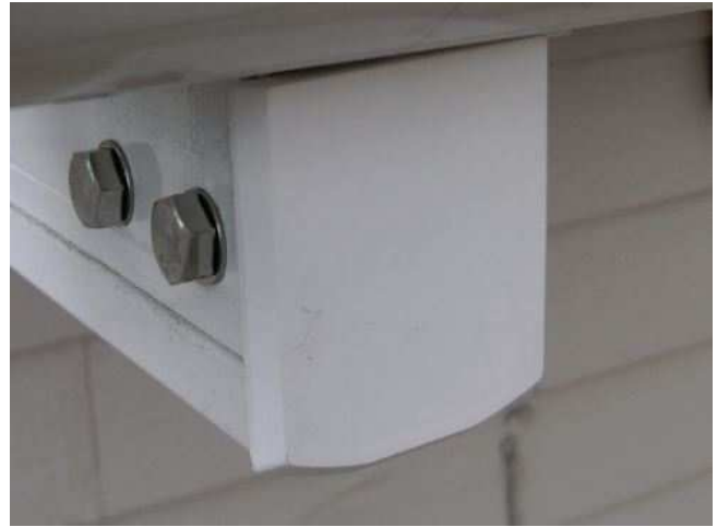
11. Install projection beam caps and secure each cap with 2 bolts with washers.
