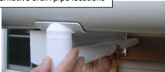
30. Select and mark the drain pipe position, on the left or right from the projection beam, with an appropriate slope toward the wall.
