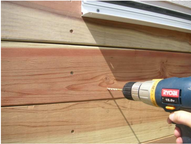
4. Drill pilot holes appropriate for the size of your fasteners.
