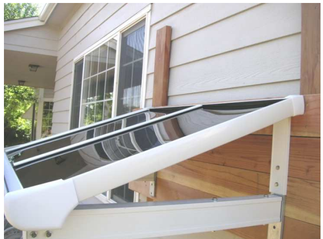
19. Apply caulk along the inside edge of the gutter (see Step 12). Install the right edge rafter with front and back caps.
