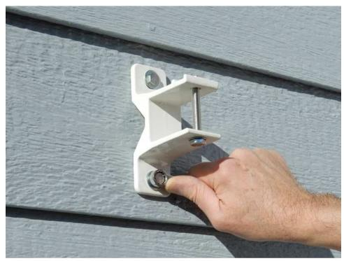
Proceed to install remaining wall brackets. The number of brackets depends on the width of your awning. Make sure that the brackets are installed on the same level and square to the ground.
