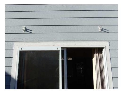
Lift the awning and insert the square bar into the brackets. You will need one or more helpers, depending on the size and weight of your awning. Secure the square bar in each bracket with the included bolt and nut. The bolt is inserted from the bottom, the nut goes on top. Tighten the bolt.
