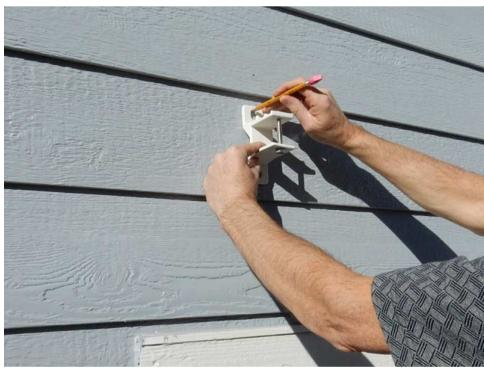
Attach the first wall bracket with two anchor screws with washers. It is the responsibility of the installer to use wall anchors appropriate for the siding and wall construction and drive them to a sufficient depth into structural elements of the building.
